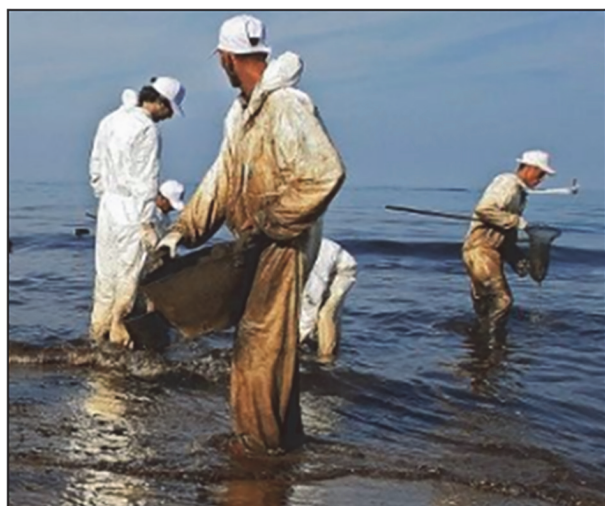
Left: Recovery of sunken oil with nets (Bernard Fichaut, University of Brest).
