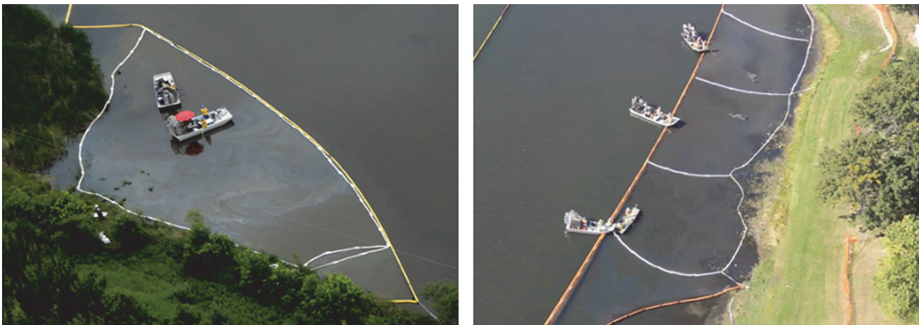
Figure 5-12—Agitation of Sediments in the Kalamazoo River Liberating Sunken Oil to Float to the Surface for Recovery (USEPA)
