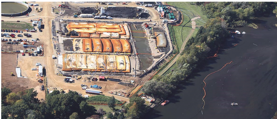
Figure 5-3—Area for Dewatering, Solids Handling, and Water Treatment During Dredging Operations in the Kalamazoo River ( www.enbridge.com )
