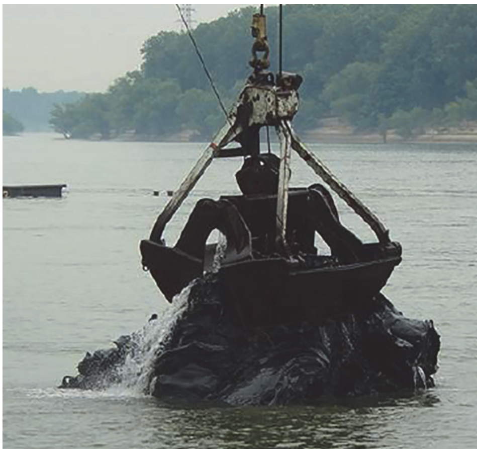
Figure 5-8—Mechanical Dredge Bucket Removing Asphalt During the T/B MM-53 (USCG)
