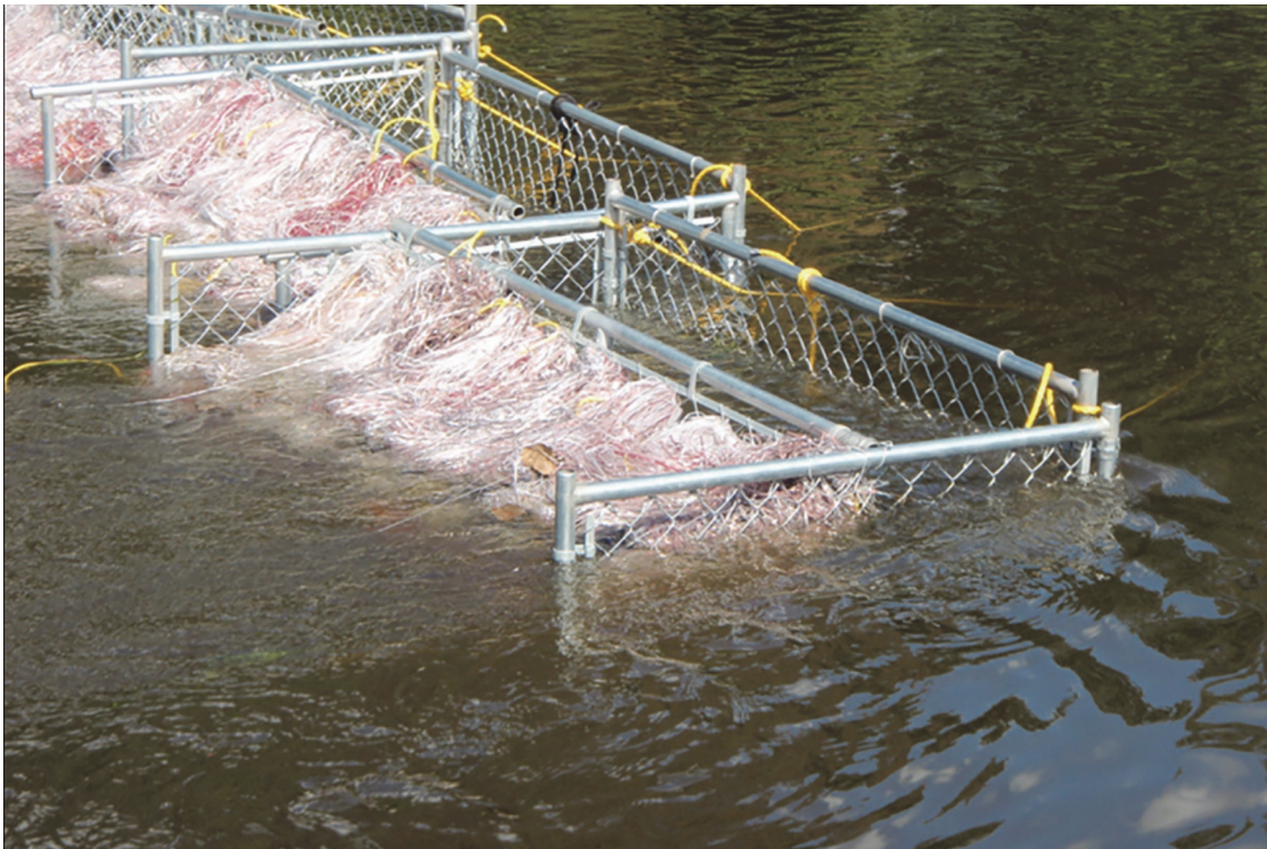
Figure 4-1—Gabion Baskets in the Kalamazoo River at the Enbridge Pipeline Spill (USEPA)
