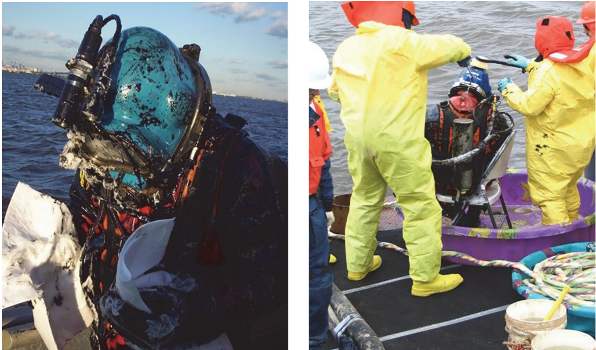
Figure 3-4—Contamination of Divers and the Decontamination Process (Elliott, 2004)
